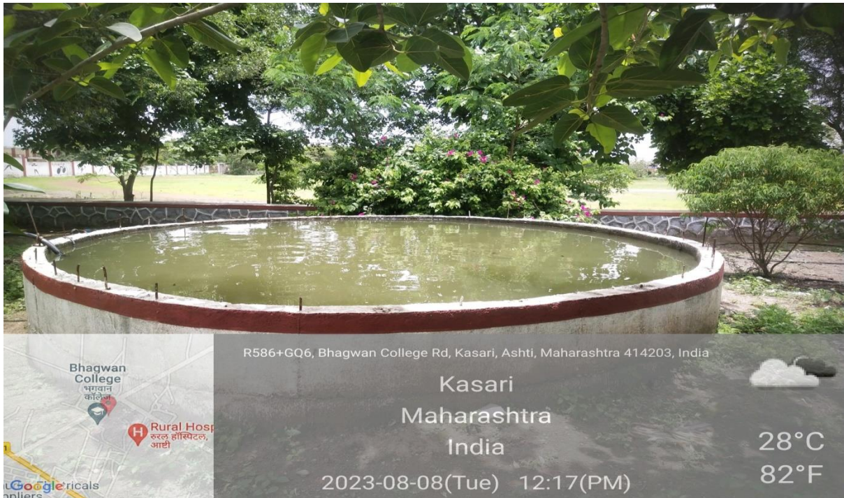
Water Tank for Tree irrigation having Capacity 50000Lit.
